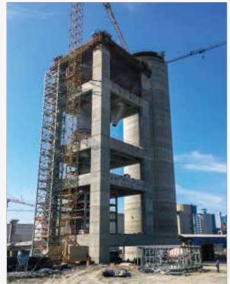
Concrete Pumping at 175 m Height
