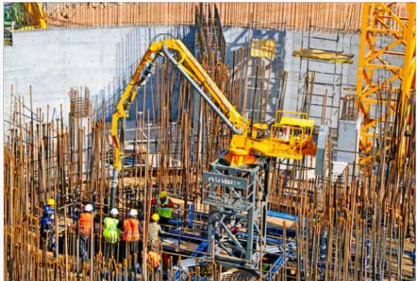
Short-Outriggers with Ballast Weights (Freestanding)
